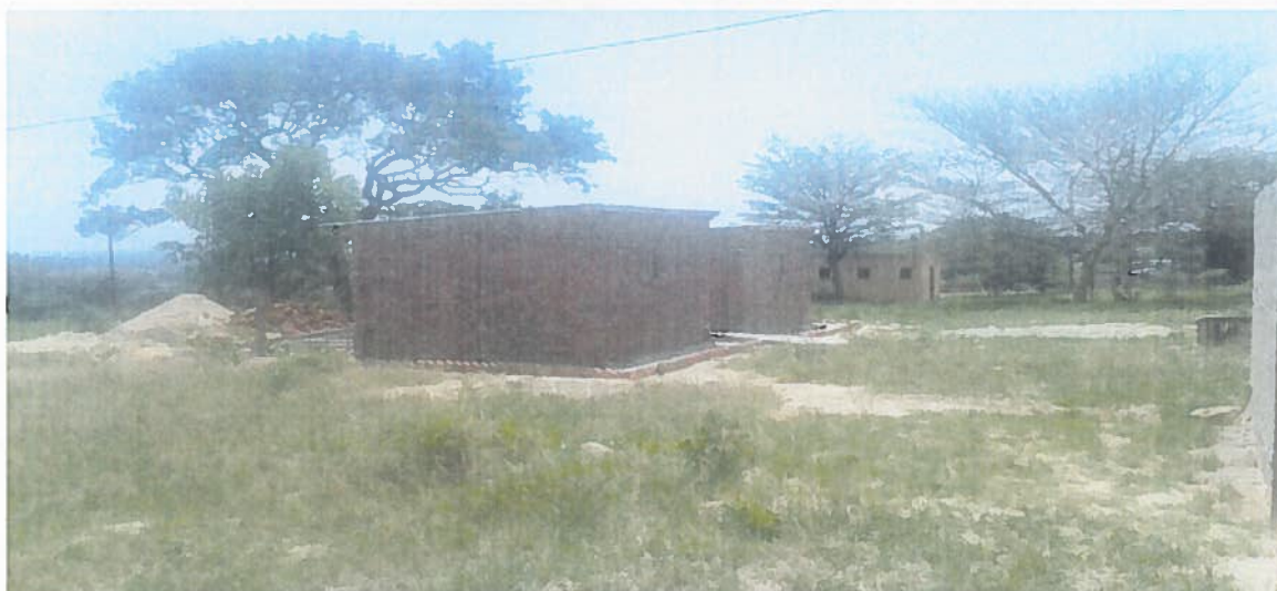
The learners' toilets constructed by the SGB
