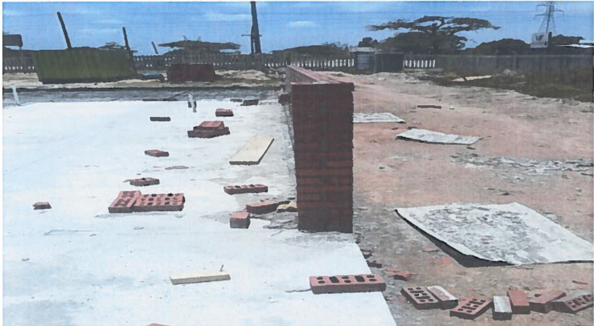
The sub-structure of the library, awaiting installation of the SIP's
